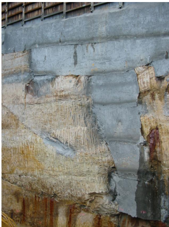
Figure 3: Example of Shotcrete Protection of Pittman LIV Dyke at Excavation Face
